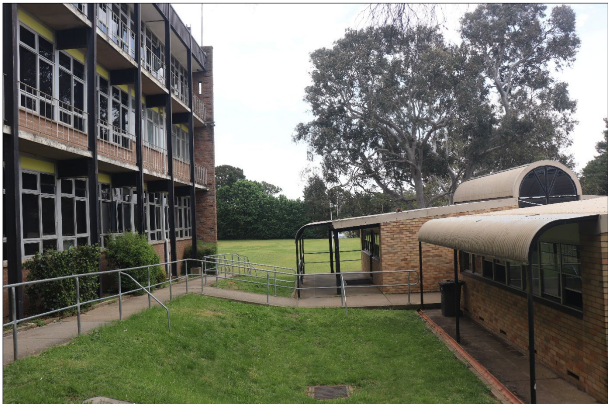
Figure 17 Relationship between the subject building and Metcalfe building adjacent
