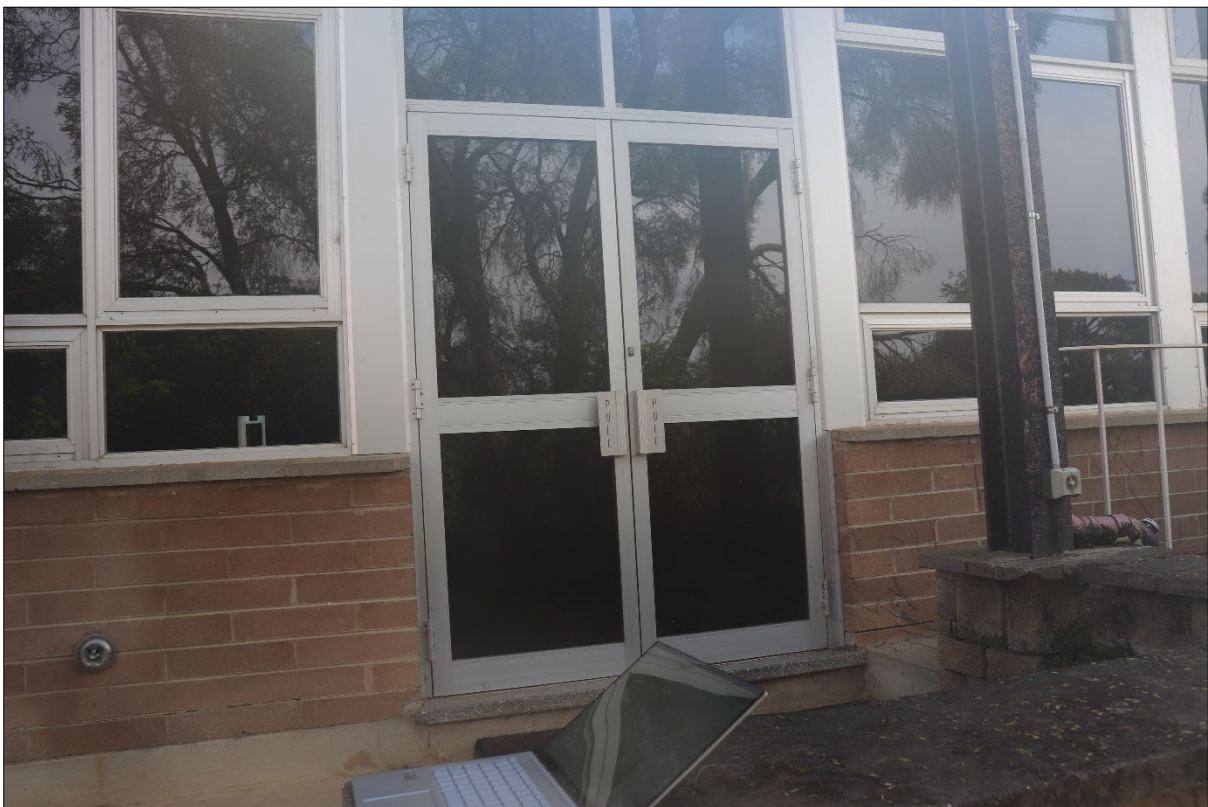
Figure 14 Connection point of new building to Metcalfe building
