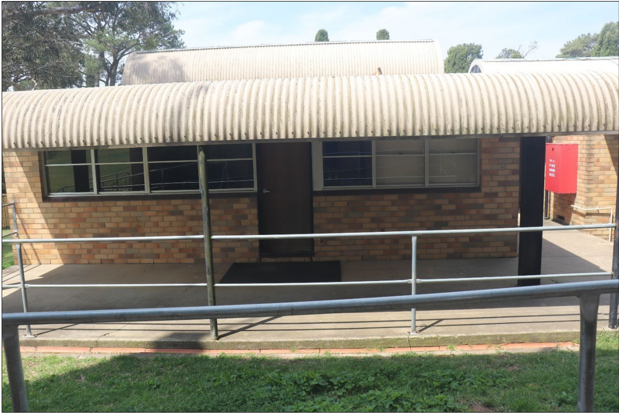
Figure 10 External view of subject building
